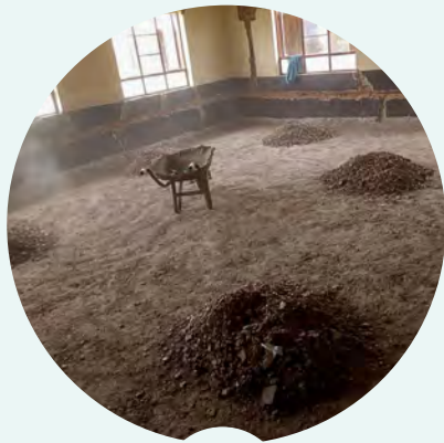
Mid-Renovation at St. Joan Academy
