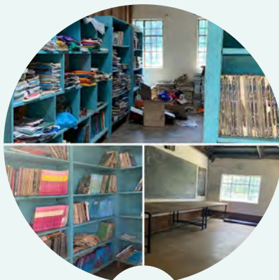
Kimwarer Secondary Library Before Renovations
